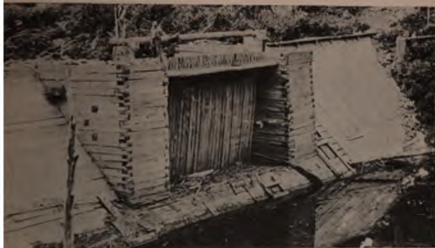
FIG. 103. — Upstream View of a Rafter Dam, showing a Needle Gate. Appalachians.
